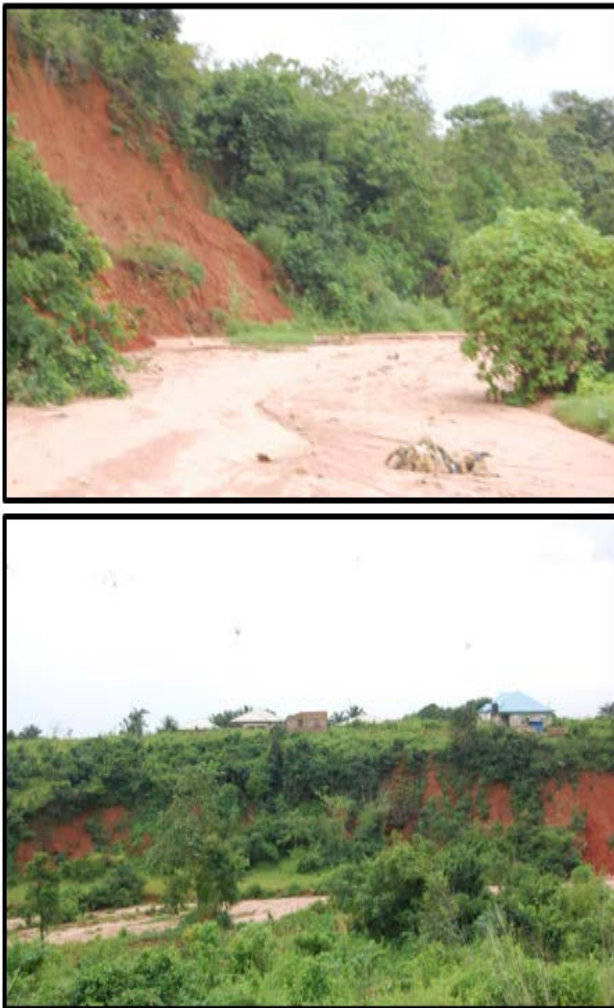
Figure 1. Some landslide locations in Ebem community, Ohafia
