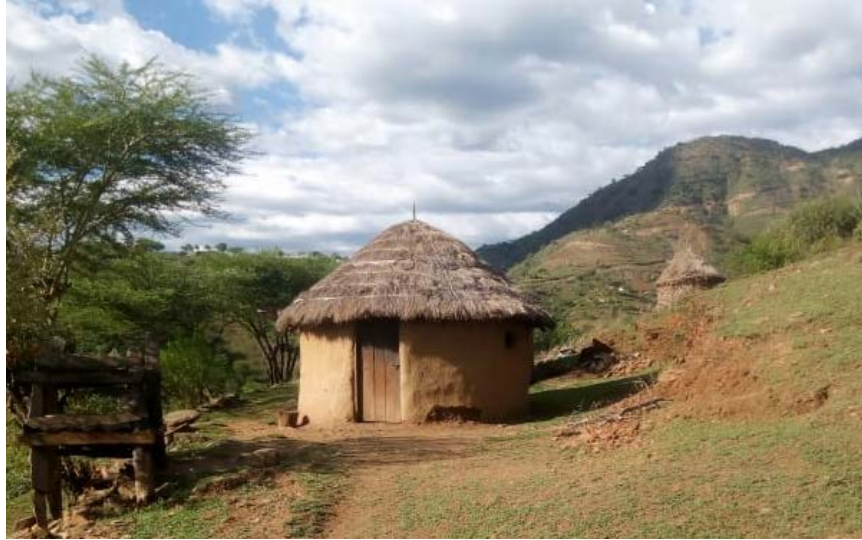
Figure 2. Photograph of mud walled houses with grass roofing
