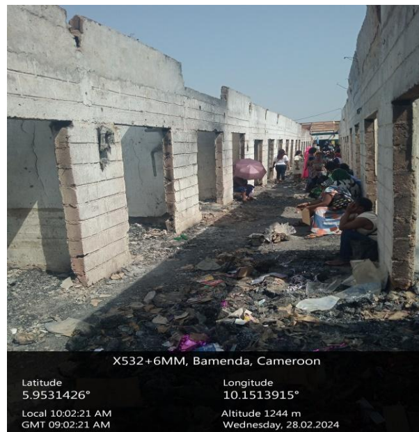
Figure 3. Insufficient spacing separating shop buildings in the Bamenda Central market
