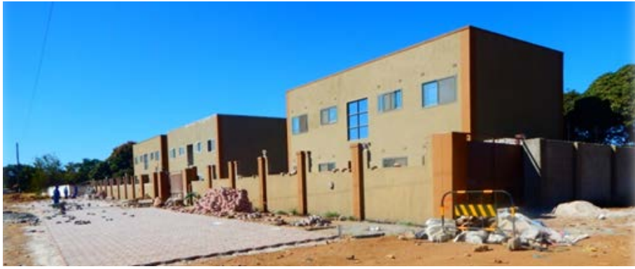
Figure 5. Apartments constructed on access road in Libala Township
