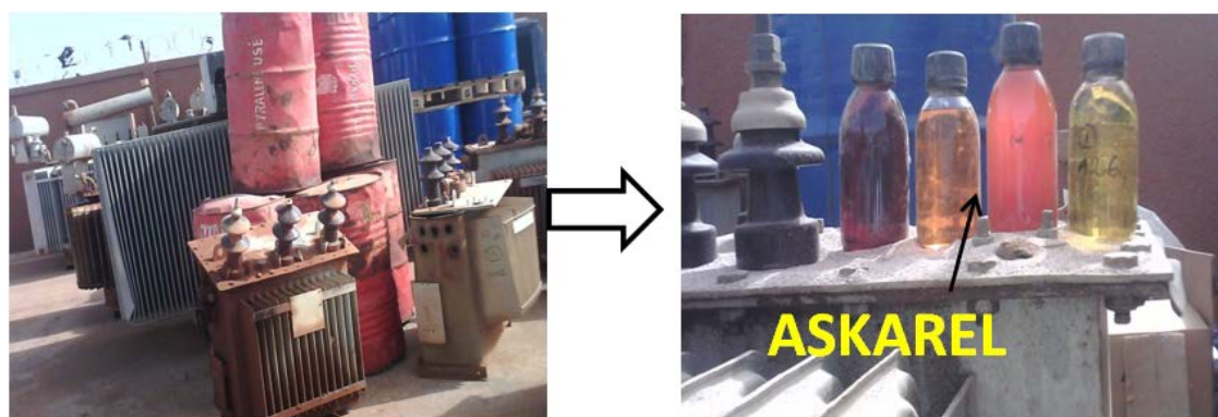
Figure 1. (a) used transformers and drums used for storing solid waste contaminated with pyralene (b) transformer oil samples with Askarel
