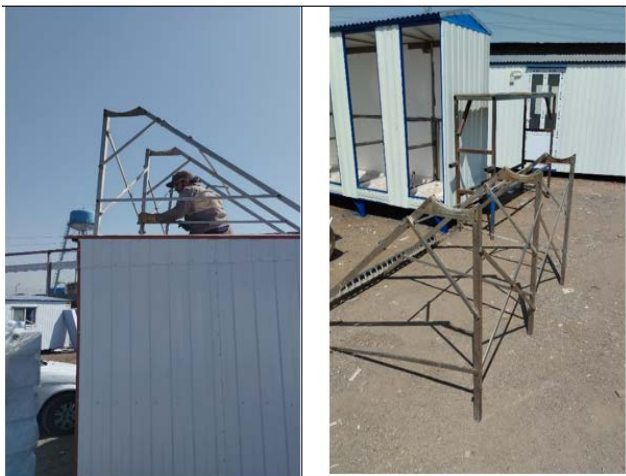
Figure 6. solar water heater installation
