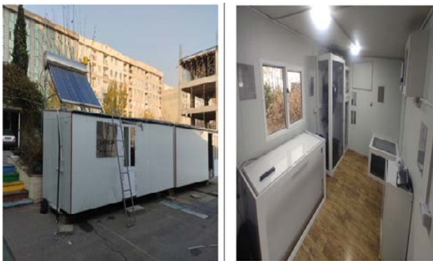
Figure 8. The interior and exterior of the portable energy booths
