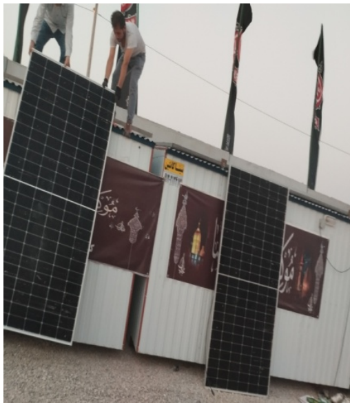
Figure 5. solar power plant installation
