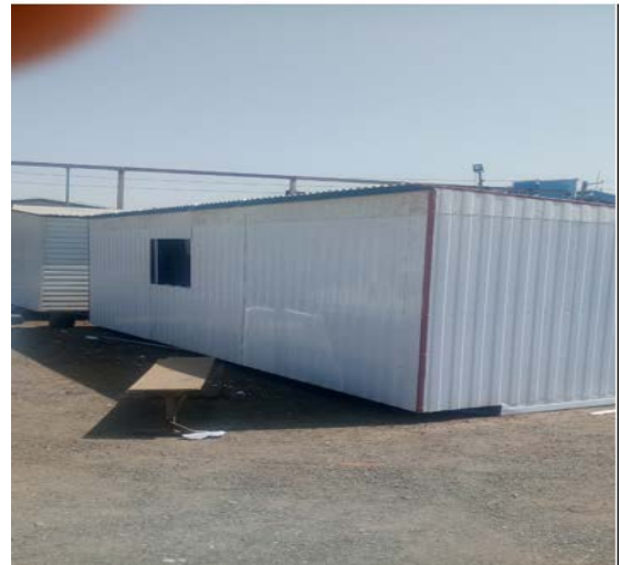
Figure 4. booths construction stages
