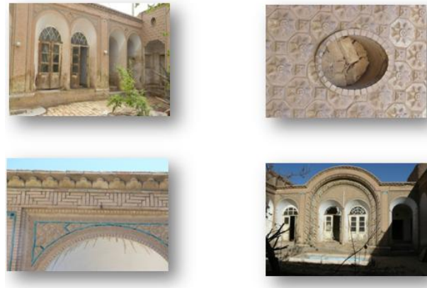
Figure 4. Module in the façade of Nikandish House
