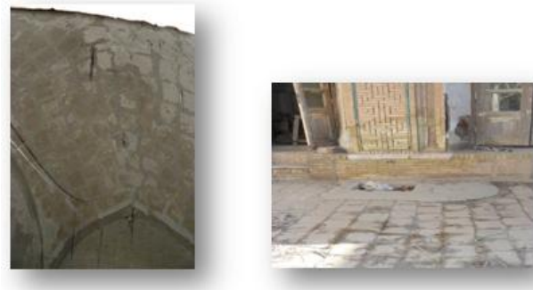
Figure 6. Using 25x25 cm bricks in yard tiling and roofs
