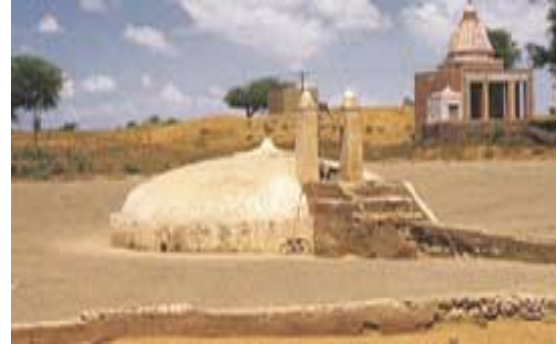
Figure 2. Underground water storage system
