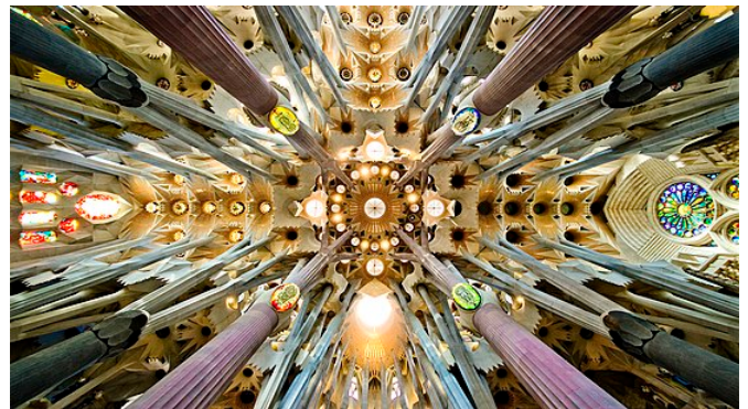
Figure 3. Sagrada Familia nave roof
