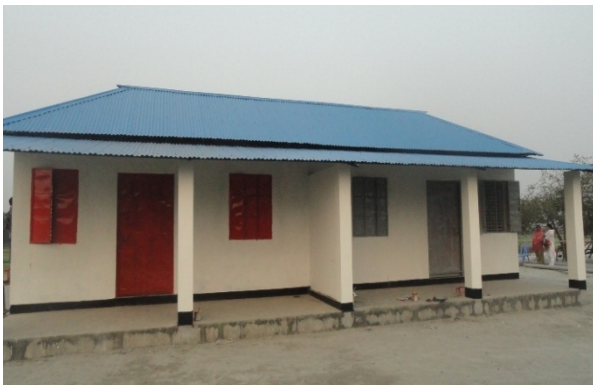
Figure 1. Resettlement house of two units (Source: Author)
