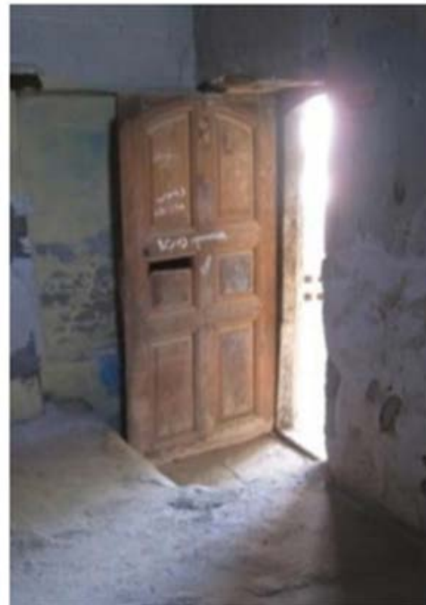
Figure 8. Level difference in rooms in historical houses ( http://www.erbilcitadel.org/ )
