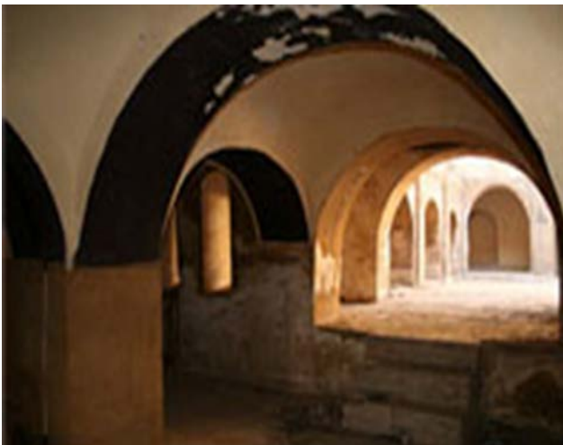
Figure 4. Semi-basement in Erbil traditional residence ( http://www.erbilcitadel.org/ )
