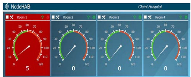
Figure 15b. Nurse Station Monitoring Screen at Alarm Case
