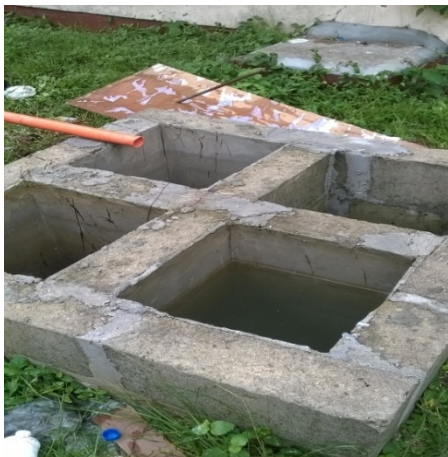
Figure 1. The constructed four chambers
