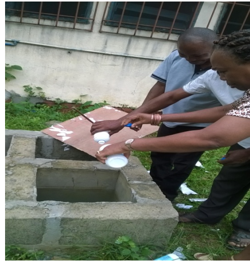
Figure 2. Filling the cathode chamber with hypochlorite solution
