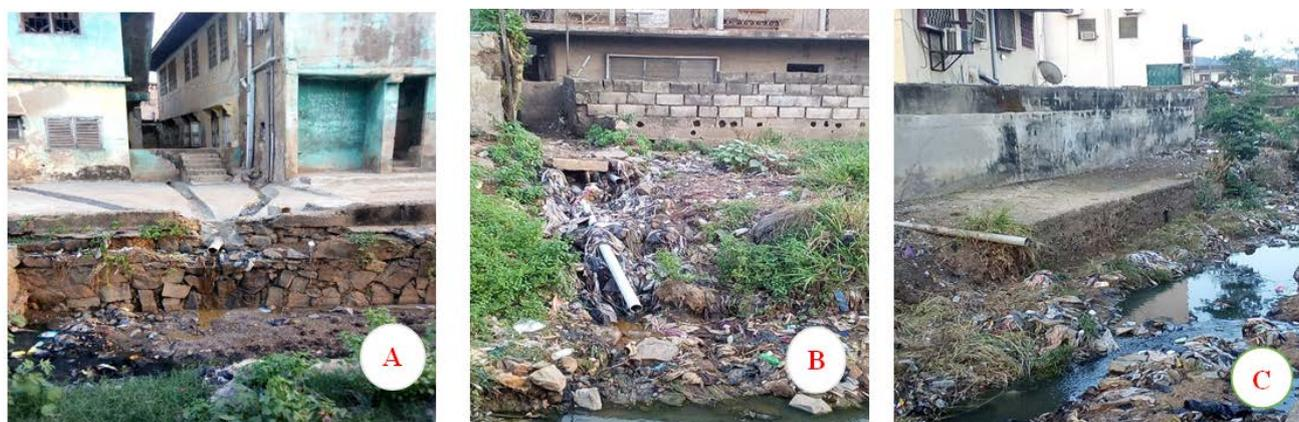
Plate 1. Plate showing faecal discharge into the nearby stream. [A: Faecal Discharge from neighbouring household into Yemetu stream, B: Pipe connected from household toilet to Yemetu stream, C: Discharge of faeces into Yemetu stream from houses that lack septic tank]
