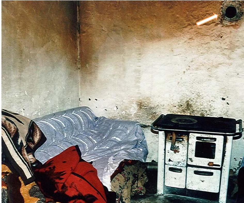
**Figure 1.** Internal view of the kitchen. The wood stove had an internal part of the tube serving as a connector with the chimney (the black hole in the right-above part of the image, **arrow**). Consider the blast effects that interrupted the tube carrying off the smoke, with fragments of blackened walls
