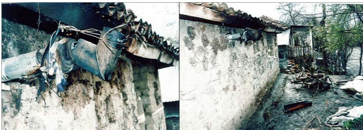
**Figure 2.** Aftermath of the lightning strike, with the burning of the external part of the chimney tube coming out from the wall (**left part of the figure**), and carbonized parts of the latter found on the ground nearby (**right part of the figure**)
