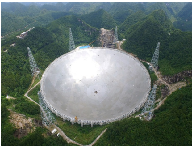
Figure 3. FAST Radio Telescope (500 m cable-suspended robot) in China ( http://fast.bao.ac.cn/en/FAST.html )
