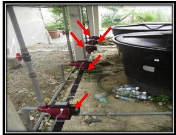
Figure 2. Water pumps (as indicated) that connected from microcontroller
