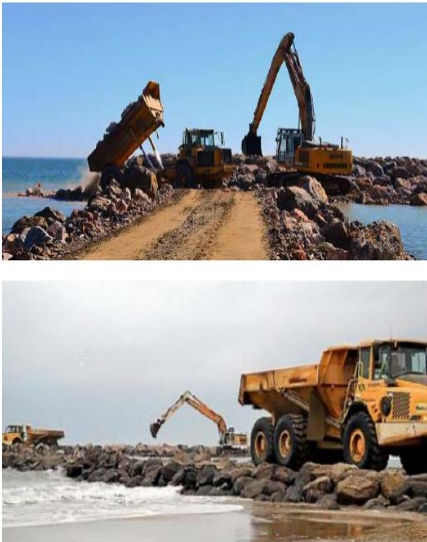
Figure 6. Laying blocks of laterites
