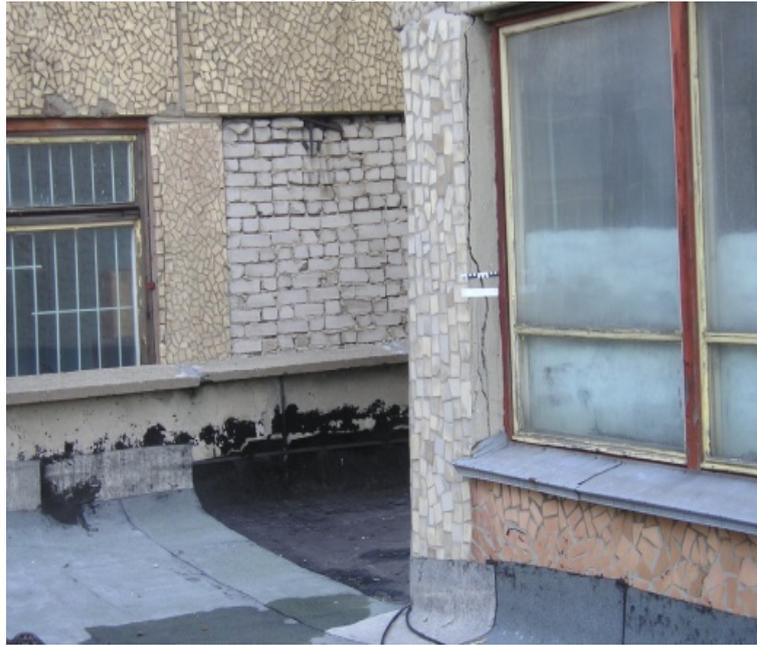
**Figure 3.** Typical crack (place of maximum stress) formed under the impact of seismic waves from large-scale blast on mines
