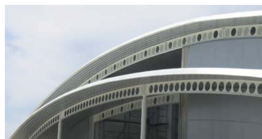
Figure 3. Construction of roofs using castellated beams
