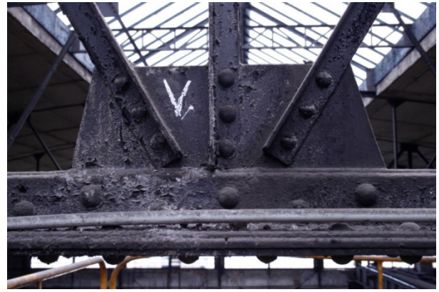
Figure 4. Riveted connection of the rods
