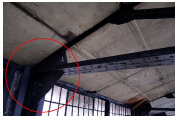
Figure 2. Supporting steel pillars of the steel roof structure
