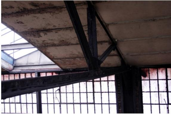
Figure 3. Rods formed by pair of L profiles
