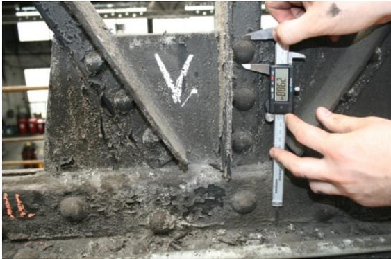
**Figure 7.** The used rivets to joining the L profiles with joint plate
