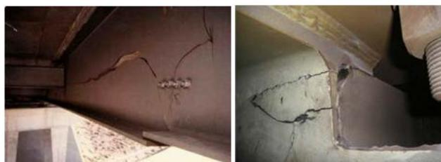
Figure 1. Cracks on beams
