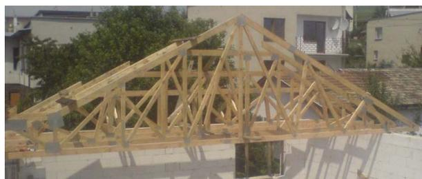
Figure 2. The truss roof structure
