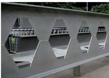
Figure 3. Bridge construction created by castellated beams [3]
