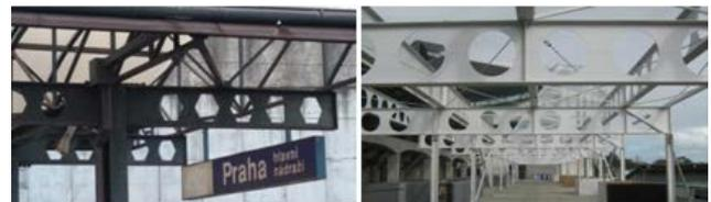
Figure 1. View of the roof structure formed from the castellated beams [2]
