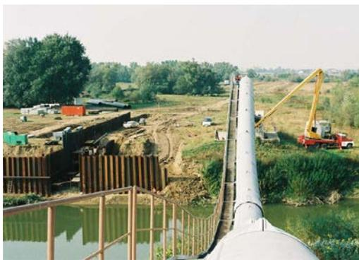
Figure 14. Existing and newly realized gas pipelines over a river flow
