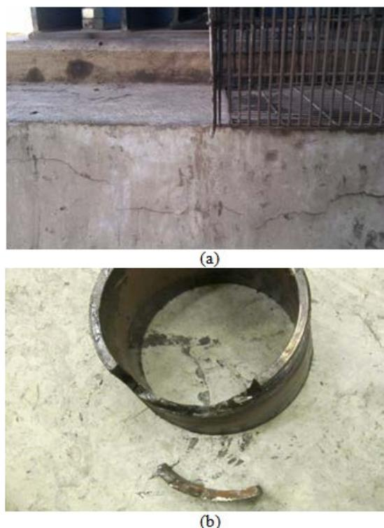
Figure 1. a) cracks in the foundation, b) damaged bearing case
