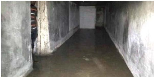
Figure 11. Ponding extends to basement corridor and room
