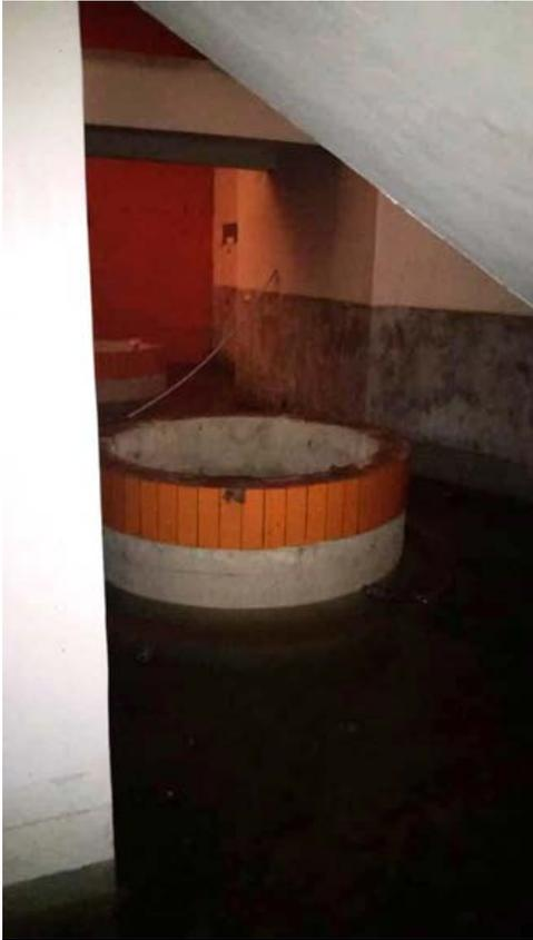
**Figure 5.** View from under the staircase showing one of the decommissioned water fountains (darker water mark below the unpainted area shows height of water usually attained overnight during flood season before pumping)
