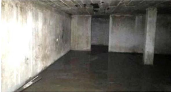
Figure 9. Water ponding on basement floor
