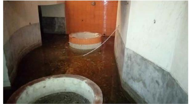
**Figure 7.** Flooded basement with water mark on wall
