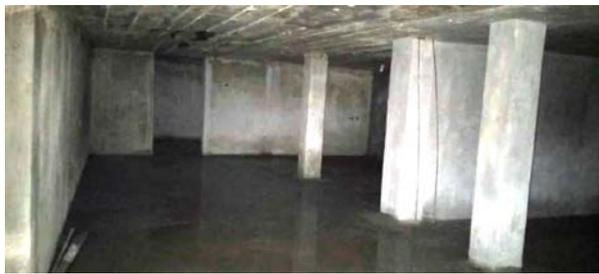
Figure 10. Showing ponding in open plan areas of the basement floor
