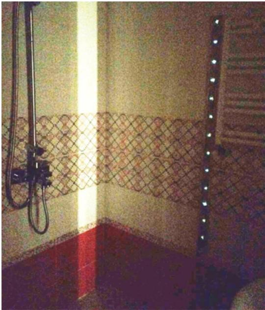
**Figure 6.** Lightening bathroom with natural light by sunlight conducting device
