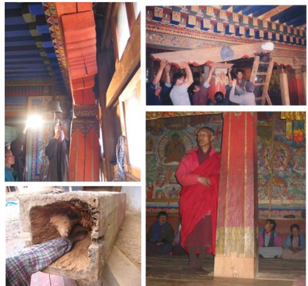
**Figure 4.** Conservation of Kachens of the upper floors. A. Condition of Kachen before intervention. B. Removal of the Kachen. C. Condition of the base of the Kachen. D. Kachen after conservation
