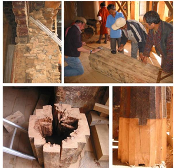
**Figure 3.** Conservation of Kachen of the ground floor. A. Kachen found embedded inside the stone wall. B. Inspection of the Kachen. C. Condition of the base of the Kachen. D. Kachen after conservation
