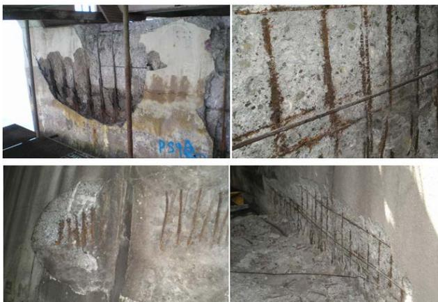
**Figure 3.** Deterioration of beams and destruction of concrete cover in a structure situated in the Persian Gulf
