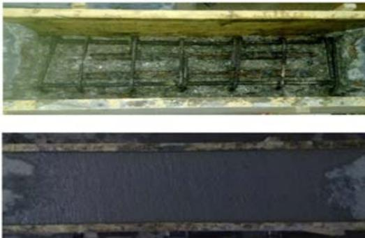
Figure 6. Photo of corroded PT beam before and after repairing
