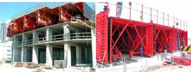
Figure 5. Tunnel Formwork System
