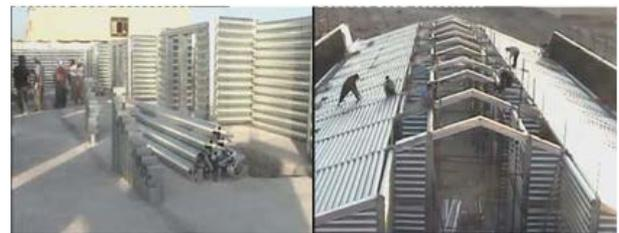
Figure 6. Tronco System using Galvanized Steel Pipe Elements
