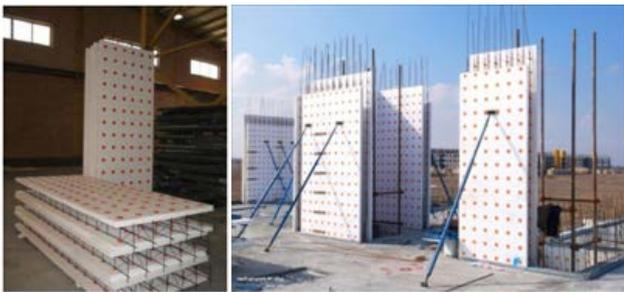
Figure 4. Preparing Insulating Concrete Formwork (ICF)
