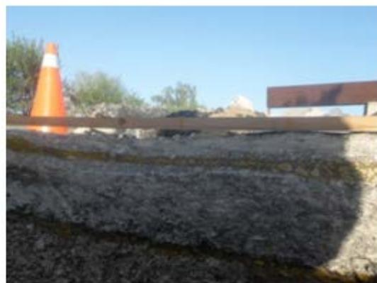
(b) HMA Failure in Right Wheel Path
