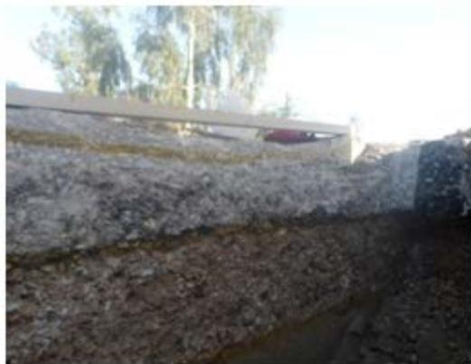
(a) HMA Failure in Left Wheel Path
