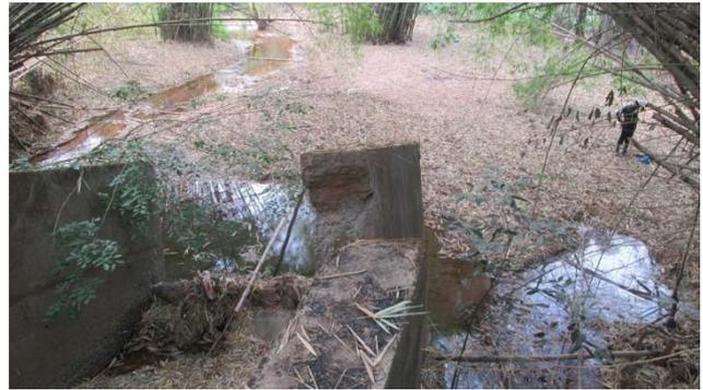
**Plate 1.** Spring flowing out from a gully in Amucha, plate also shows destroyed engineering structure used for gully control. Gully head situated behind the camera, hence not visible in plate
