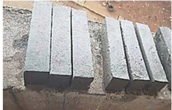
Figure 9. Demolding after 24 Hours
